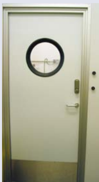
Figure 4: This door is the restricted access to the clean room for making up MDV vaccine for administration. The room is under positive pressure with air filtration.
